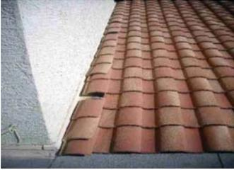
We observed roof tile(s) that are cut so that the material under the tile is exposed. Exposure to the elements can damage the material under the tile and cause roof leaks. We recommend that a qualified roofing contractor replace all improperly cut tiles. The tile(s) requiring attention include: several tiles at roof hips.
