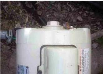
We observed that the pool timer inner cover is absent and that the outer cover is damaged. This is an electrical shock safety hazard. We recommend replacement of the timer box by a qualified technician.
