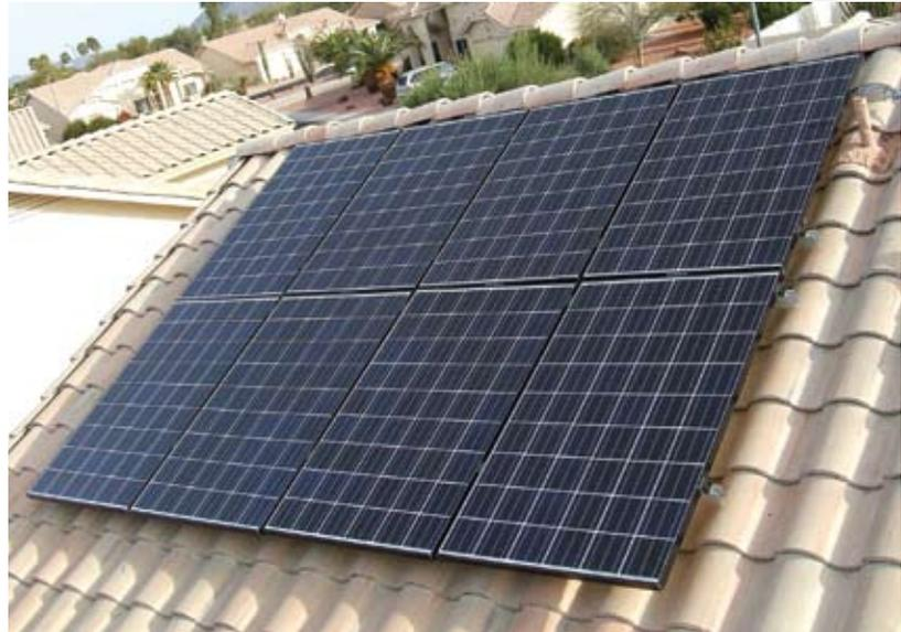
Eight PV modules are connected in an array on this roof.
